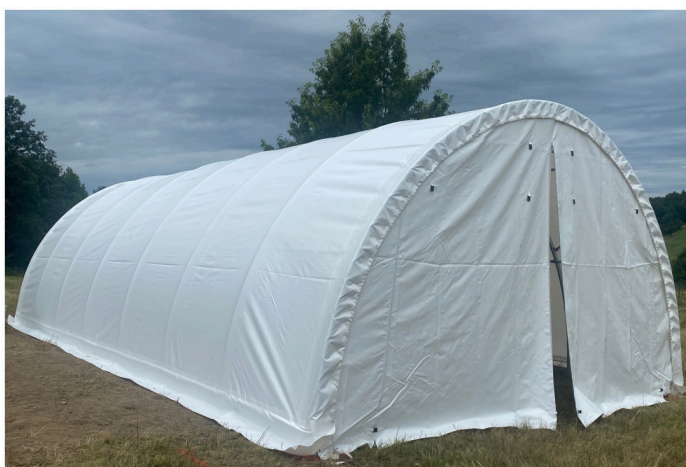
Finished tent hall
