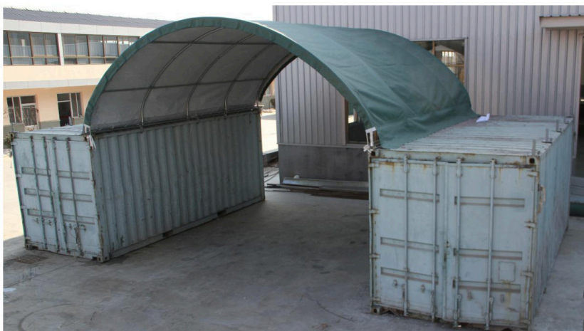
Fig. 9 – Shelter with roof cover
